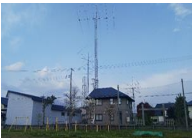
KAZU's home and towers.
