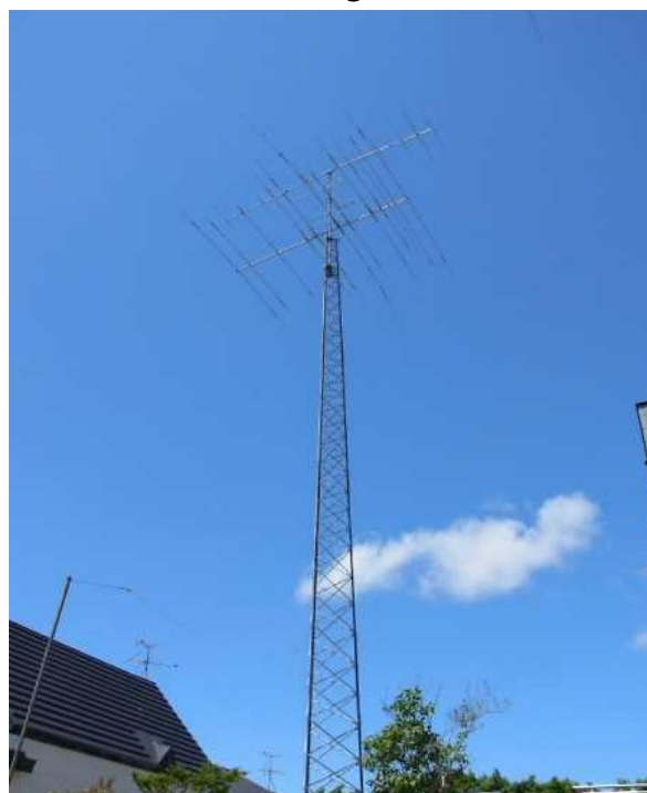
Top to bottom: 50MHz 8 ele Yagi, 430MHz Yagi stack, 7-28 MHz 12 ele Yagi, 1.9 MHz long wire(barely visible)
